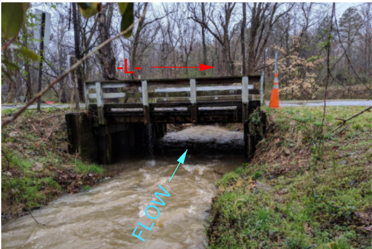
LOOKING DOWNSTREAM TOWARD BRIDGE NO. 459
